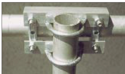
Figure 17: Mechanical realisation of the connection points for pipes for an H-shaped cross with aluminium brackets Photos: DK7ZB
